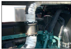
Compensatore gas di scarico Exhaust gas compensator Compensateur d'échappement Junta flexible para escape
