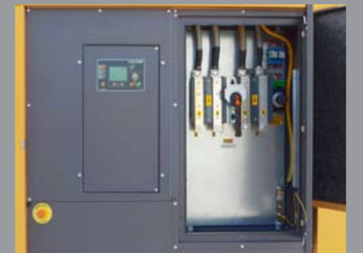
QPE-C-VCC (variant +010) Automatic panel with switching on board
